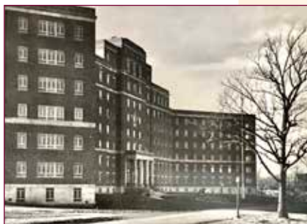
Figure 5. Providence V.A. Hospital, 1948. [NATIONAL REGISTER OF HISTORIC PLACES 1 ]
